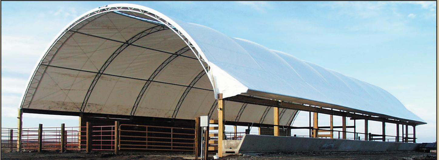
An alternative to open feedlots where runoff and manure management are a growing concern, hoop barns are considered a more environmentally friendly option to traditional open feedlot arrangements. Recent research has compared the hoop barn to open feedlots, as well as other housing options, in an attempt to determine its advantages. Hoop barn cattle feeding often confines the cattle inside the hoop barn and relies on bedding to maintain the animal environment.
