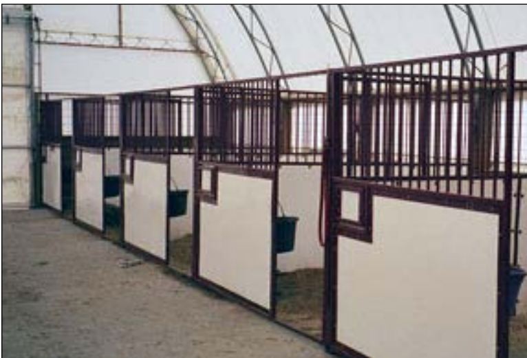
The space available in hoop barns permit a number of activities and arrangements.
